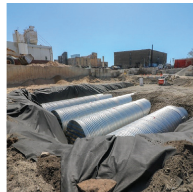
Underground rainwater cistern being installed 8
