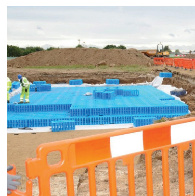
Underground infiltration crates being installed 10
