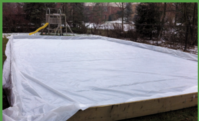
Figure 2: Building a typical backyard rink
