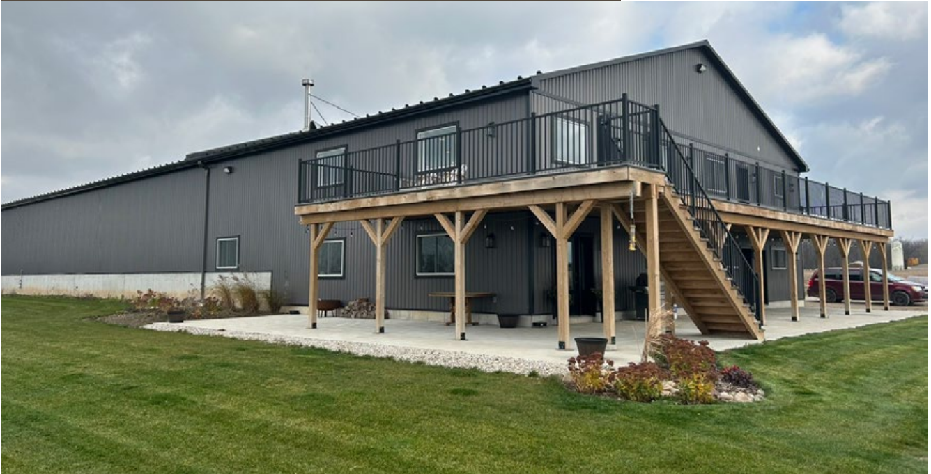
Figure 9 Recently constructed “barndominium” in Huron County
